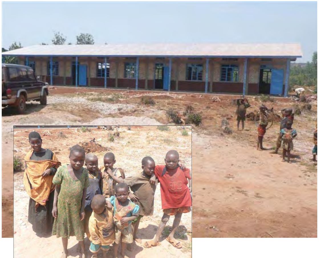
Mashitsi Village, Burundi: School construction and furniture was provided by the Benelux team.
